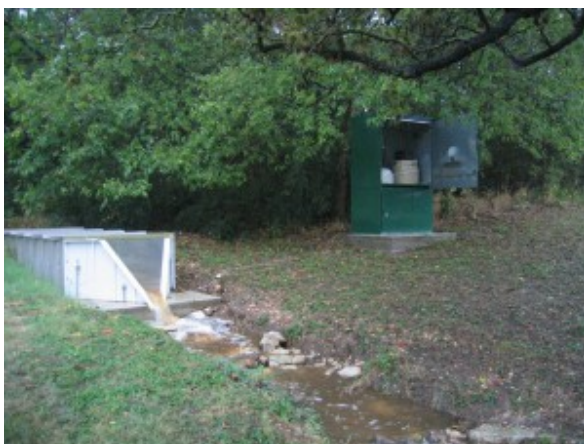
The City of Austin measures streamflow here using an H-flume. Image credit: COA-WPD-WQM
